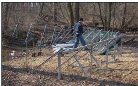
AWS Water Quality Specialist Masaya Maeda inspects placement of plastic mesh squares during construction of AWS’s new Nash Run trash trap (February 2009).
